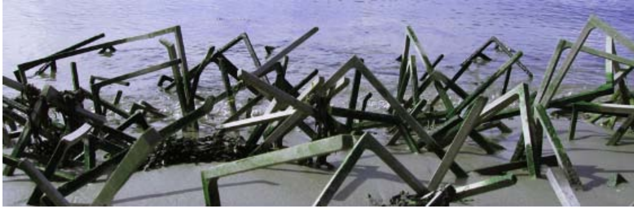
Ground consolidators for shoreline protection design by Bureau Witteveen+Bos source: www.witteveenbos.nl
